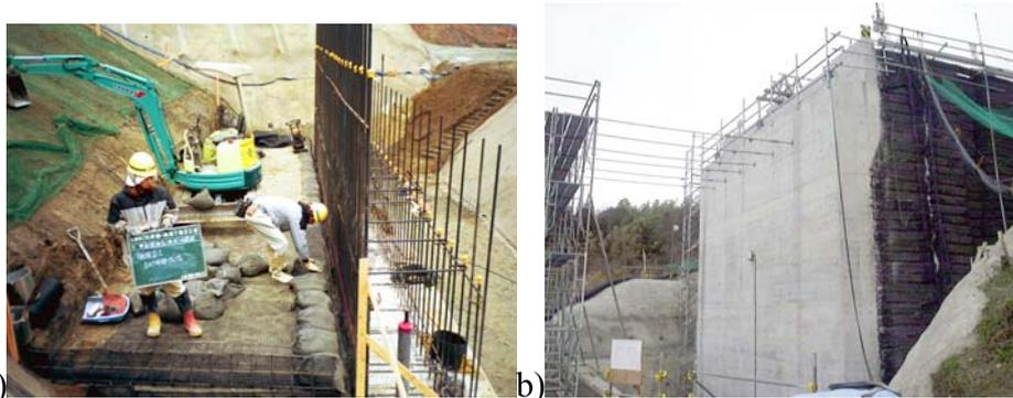
*Fig. 32 a) Placing gravel-filled bags at the shoulder of each soil layer; steel reinforcement seen in this picture is for the parapet that was constructed after the backfill was completed (Watanabe et al., 2003b); and b) bridge abutment with backfill of cement-mixed gravel during full-scale loading test.*
