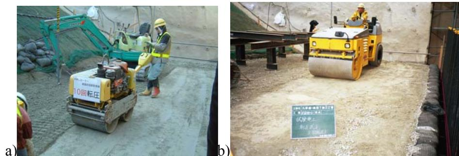
**Fig. 30** Compaction of the backfill
